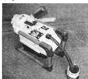
Fig.5 Blockage clearing equipment
