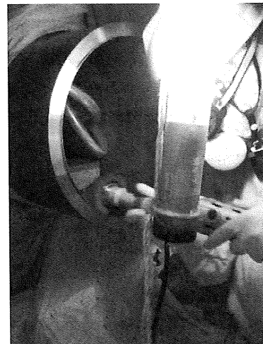
Fig.10 Polishing inside the Piping
