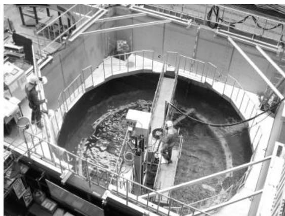
Fig. 3. WJP work situation in manufacturing factory before shipment to power plant site.
