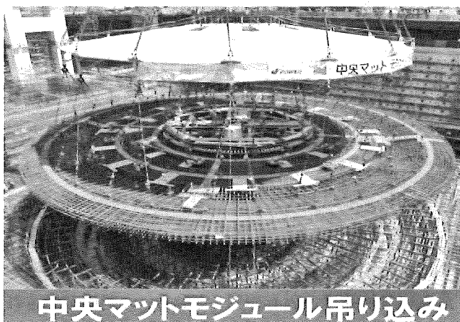
Fig.3 Reinforcing steel structure for nuclear reactor building
