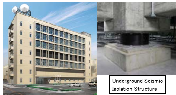
Fig.4 Office building with seismically isolated structure
