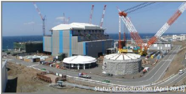
Fig.2 Location and the present condition
