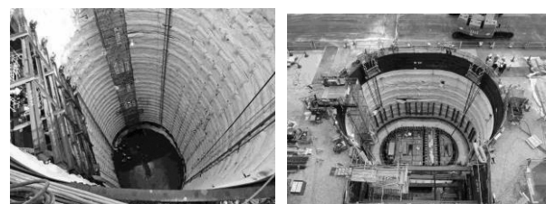
Fig.8 Construction on site (left: Sep. 2013, right: May. 2014)
