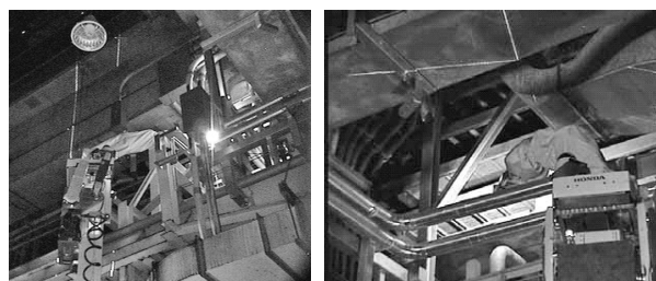
Fig.2 Surveillance Mission in Unit 2 (provided by TEPCO)
