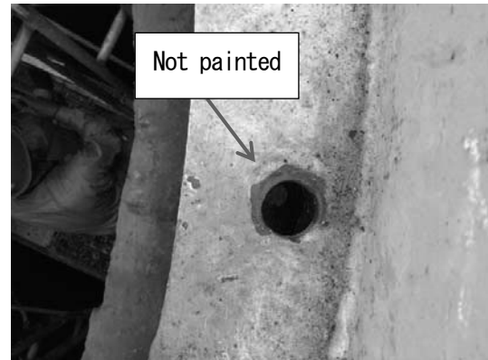
Fig. 12 Photo of flange plate and anchor bolt hole
