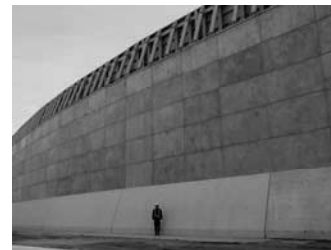
Fig.3 Tsunami protection all
