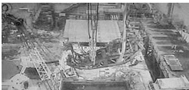
Fig.3 Fuel handling machine removal operation at site
