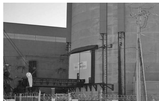
Fig.2 Decommissioning of Zion NPP
