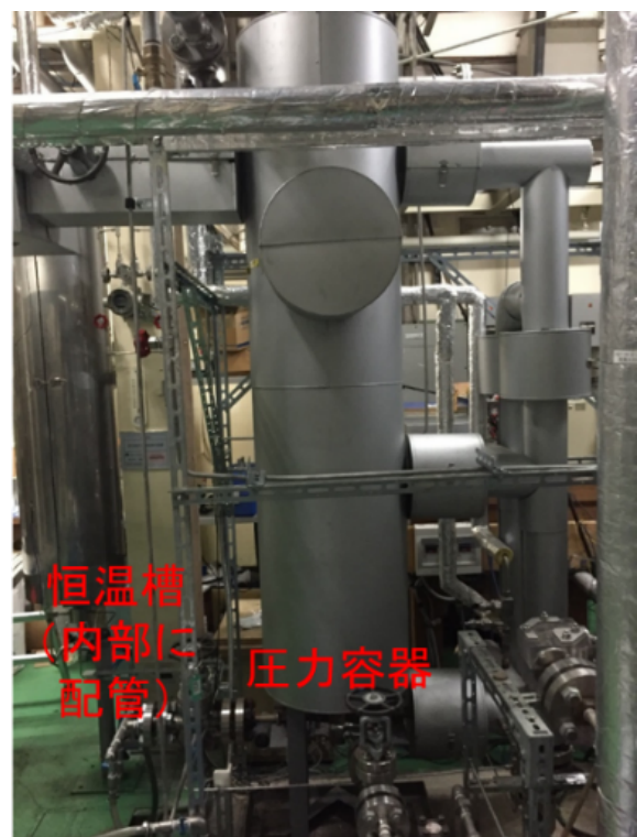
Fig. 2 Mock up test facility for back fill
