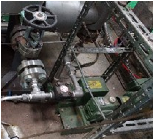
Fig.4 Plunger pump for back fill
