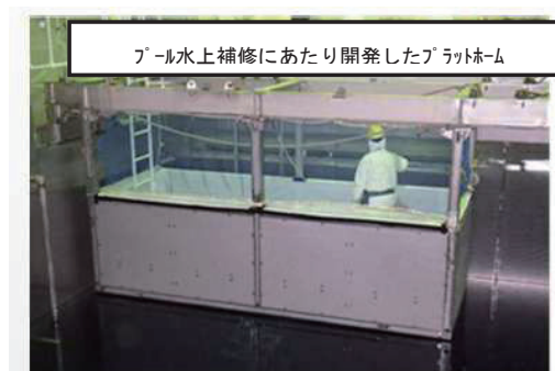
Fig.5 Work scenery of on-water repairing
