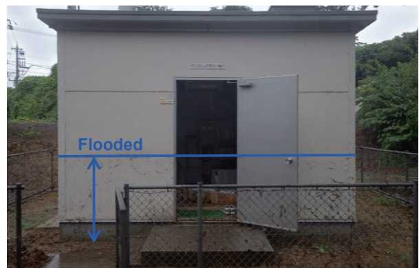
Fig.2 Situation of monitoring post No.1 was flooded
