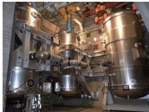
Fig.4 Installation of FCVS filter vessels
